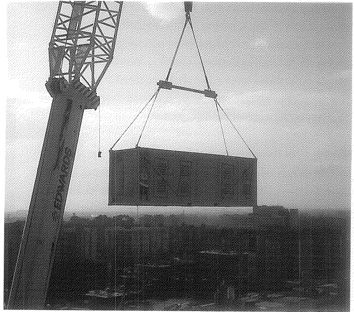
Two C800 power packages produce electrical and thermal power at this 10-story building in downtown Bogota, Colombia.
