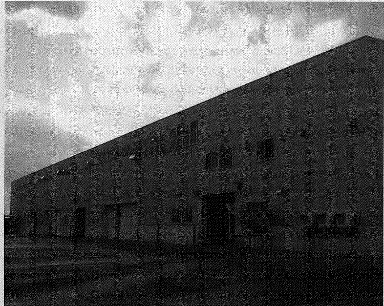
Methane gas fuels four C30 microturbines at a garbage-processing center in Japan.
