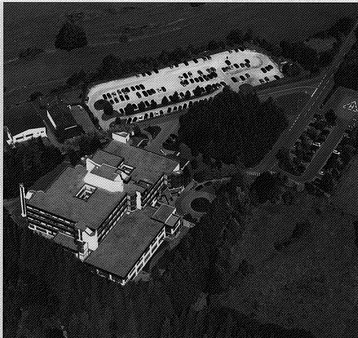
A Capstone C65 microturbine produces electrical and thermal power at St. Joseph Hospital in Germany.
