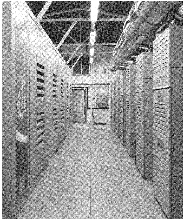
A natural gas C1000 Power Package and 10 C65 Microturbines provide all electricity and heat required by the shopping center.
