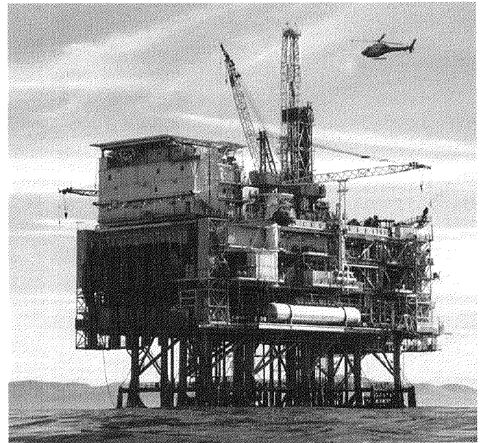
Forty six Capstone microturbines provide prime power to twenty seven offshore oil rigs in the Gulf of Mexico.
